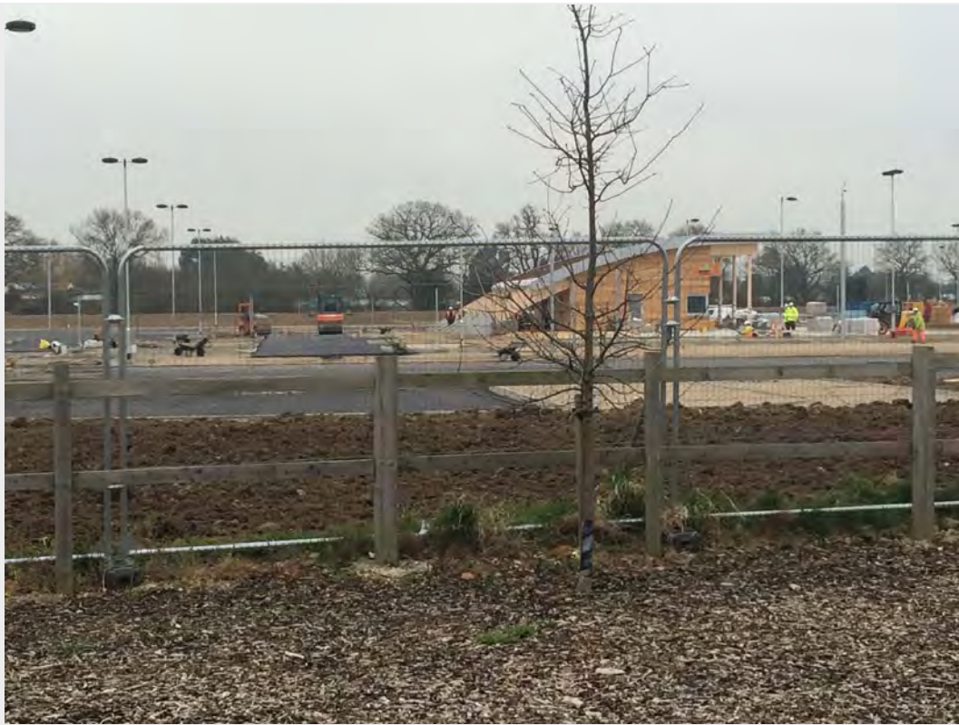
The Colchester Park and Ride site taking shape
